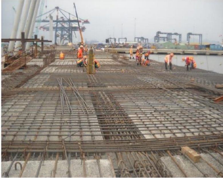
Figure 17 Deck slab construction
