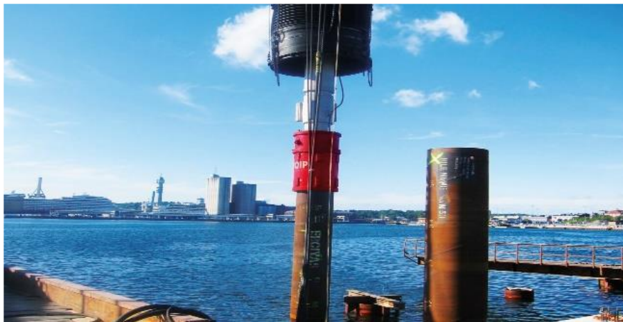
Figure 4 Hydro hammer with Noise shield
