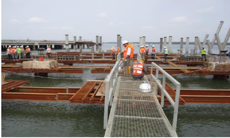
Figure 15 Pile cap concreting
